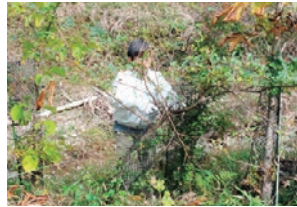
Removal of anti-deer fencing
