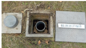
Well for automated inspection of underground water pH
