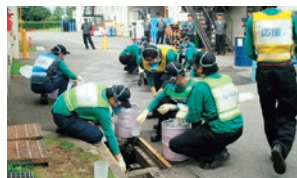
(4) Leaked liquid is recovered from the gutter area
