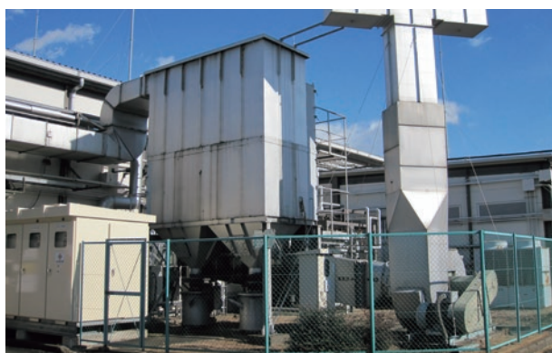
Deodorizing equipment (dust collector)
